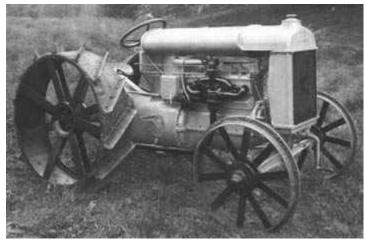
Fordson Model F 20 H.P., four cylinder engine delivered 10 H.P. on the drawbar 3 speed spur gear transmission Produced from 1917-1928 at Dearborn in America Produced from 1919-1922 at Cork, Ireland
